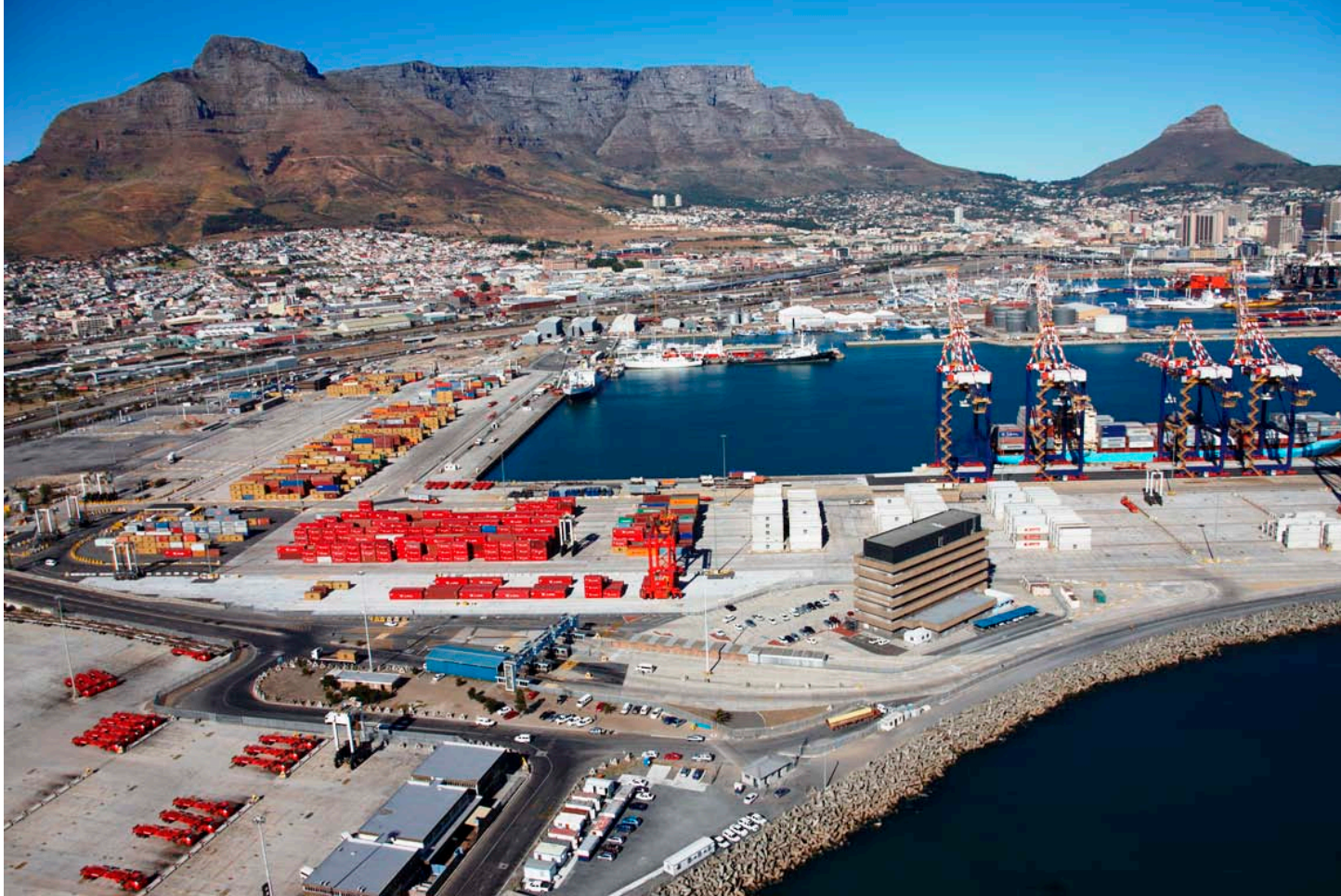
The Hatch Mott MacDonald and Goba (HMG) JV assisted Transnet in deepening the Cape Town Container Terminal's existing four berths as well as reconfiguring and modernizing the container storage yards.
